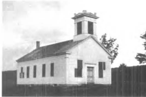
The Craftsbury Reformed Presbyterian Church, built ca. 1835 and torn down 1910. Courtesy of John Woodruff, Simpson Memorial Library, Craftsbury, Vermont.
