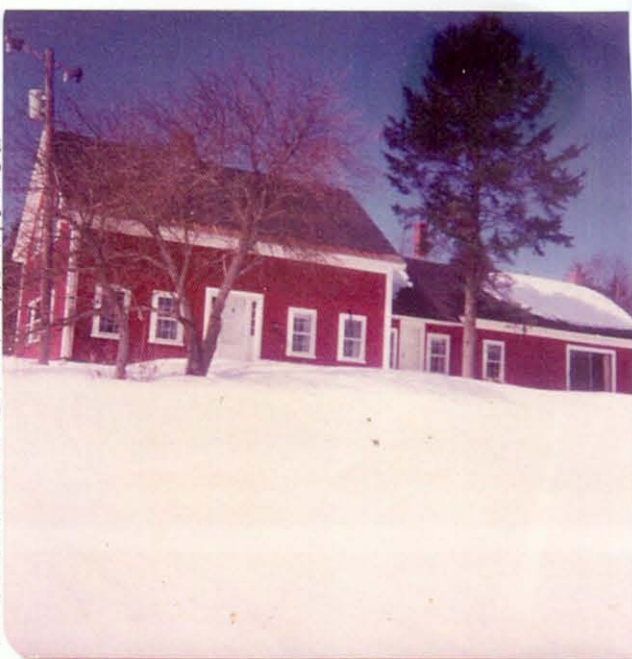
BUILT- ANDREW BARR HOUSE GREENSBORO REMODELED- STEVENS HOUSE
